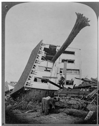
The Johnstown calamity. "A slightly damaged house."
